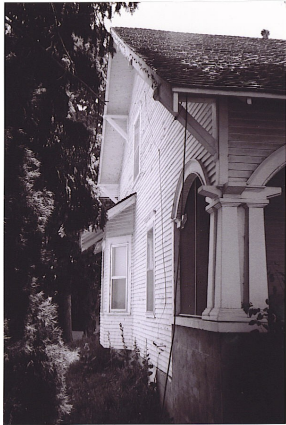
Main House: east elevation, showing bay window, view to south
